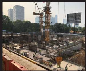
Most of the ground floor area has already been casted and next will install the rebar.
